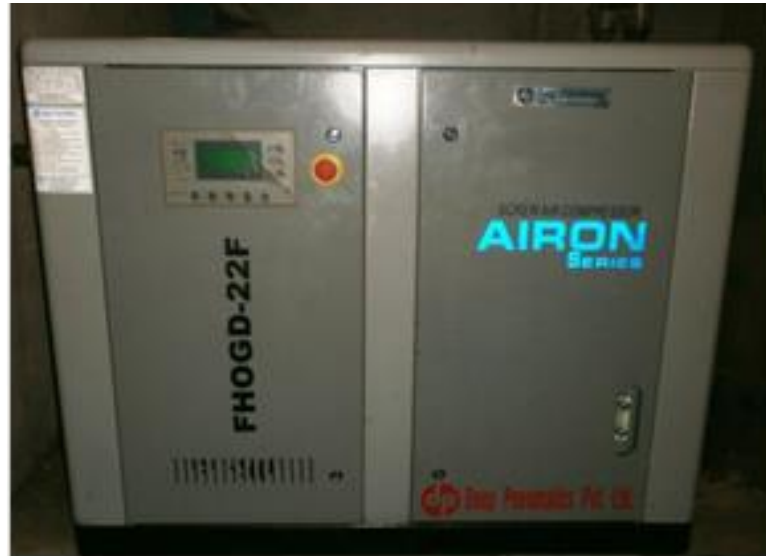
Replacing reciprocating air compressor (L) with VFD-based screw air compressor (R)
