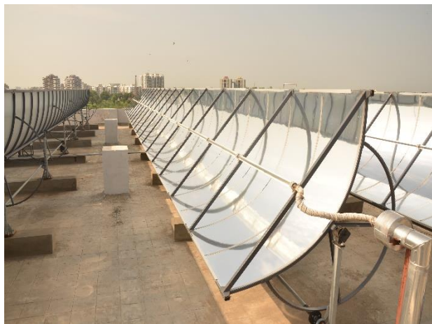
Concentrated Solar Thermal Steam Generation system
