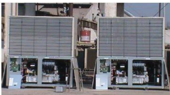
GHP system – outdoor unit (L) indoor unit (R)
