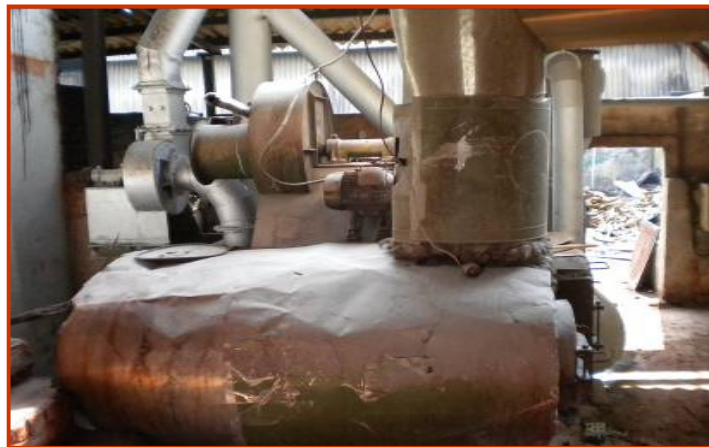
Figure 2.1 Energy efficient wood fired hot air generator
