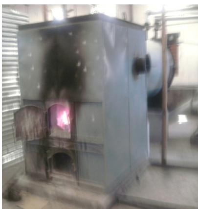
Figure 1.2 Thermic Fluid Heater
