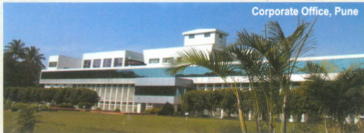
Corporate Office, Pune
