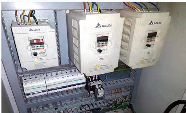
VFDs installed in motors
