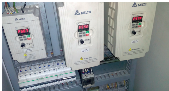
VFDs installed in cranes and hoists
