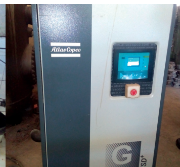
Screw compressor with VFD (in larger units)
