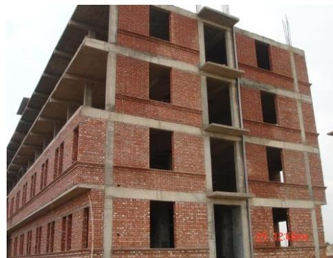
There is also a significant reduction in the consumption of top (agricultural) soil which is the main raw material in brick making. Increased use of REBs in building construction would also help in reducing the energy consumption of buildings due to their improved insulation properties.
