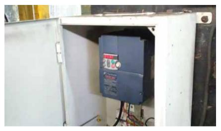
VFDs installed in cranes and hoists
