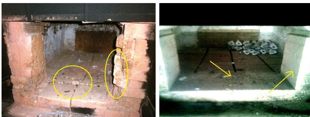
Relining shell baking furnace: (L) damaged lining; (R) repaired lining
