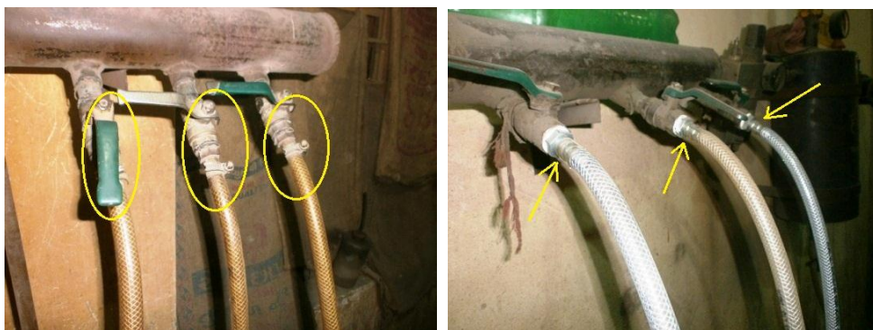
Arresting air leakages in compressed air system (L) by using crimped hose joints (R)
