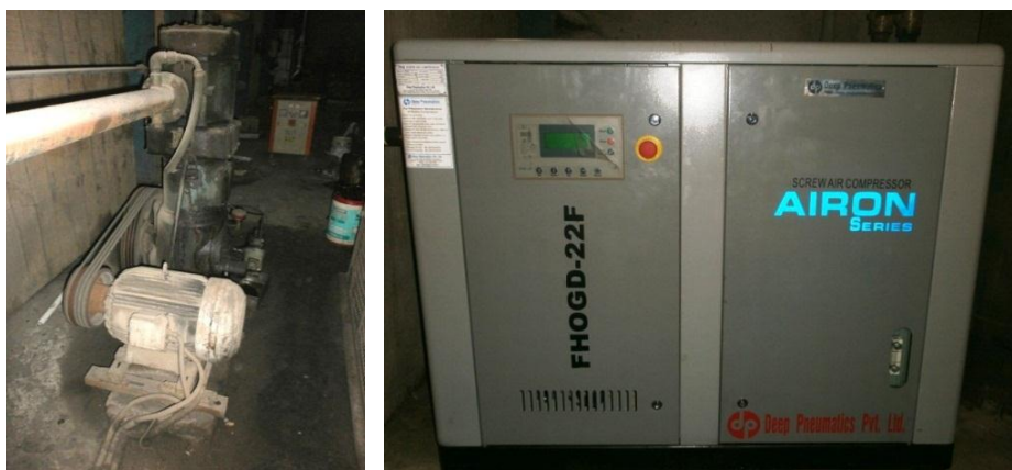
Replacing reciprocating air compressor (L) with VFD-based screw air compressor (R)
