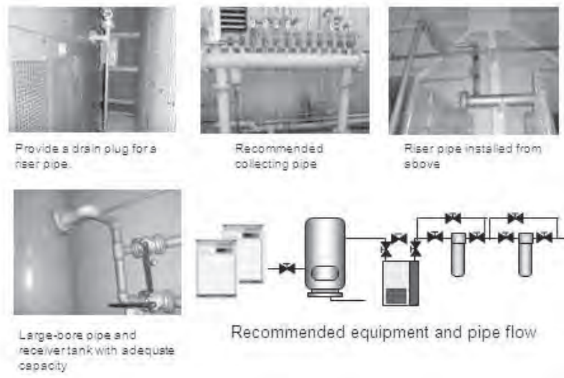
Figure 3.2.3b: Examples of recommended piping
