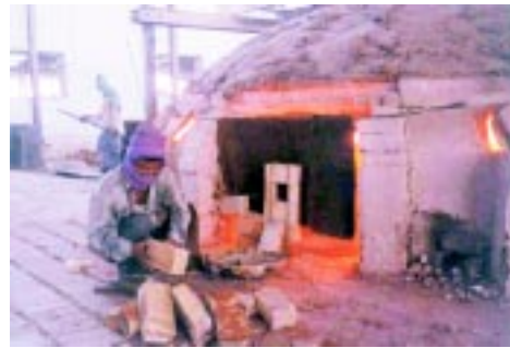
(x) Rebuilding of wall begins with placing of the centre piece
