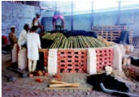
(iii) Filling the structure with mud
