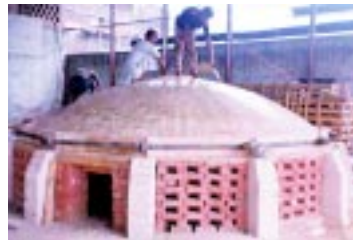
(viii) Washing the crown with silica mortar
