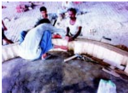
(vi) Fixing silica bricks
