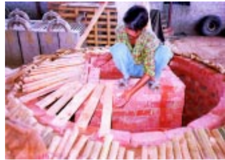
(ii) Using bamboo and planks as support
