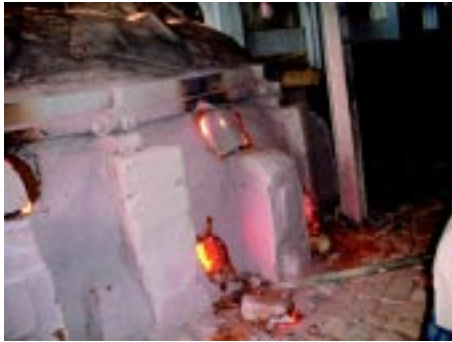
(i) Dismantling of pot furnace wall begins
