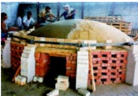
(v) Plastering the crown with mud
