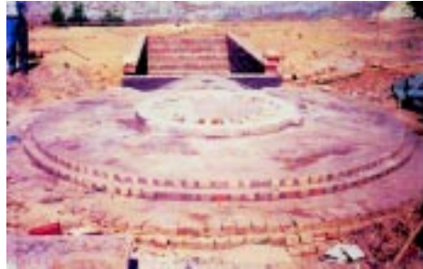
Figure 23 (Continued) Construction of base and floor
