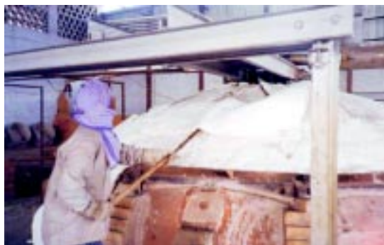
Figure 33 Ceramic fibre being laid on the crown
