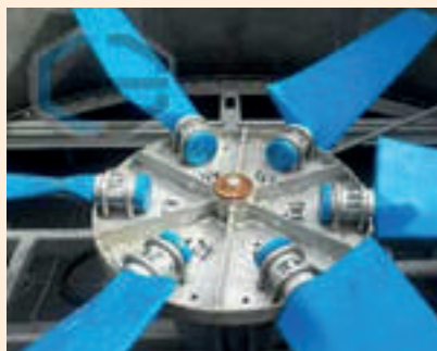
FRP fan blades for cooling towers
