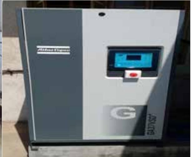
**Screw compressor with VFD**
