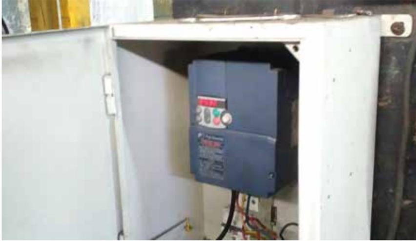
*VFDs installed in cranes and hoists*
